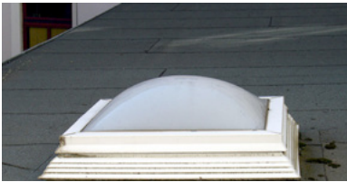
Figure 6. Sealed dome skylight
