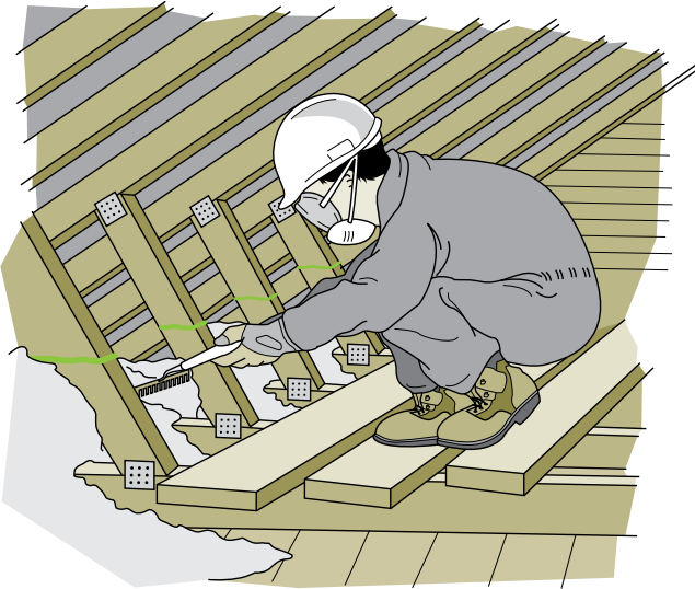
Figure 5-14 Installing loose-fill insulation
