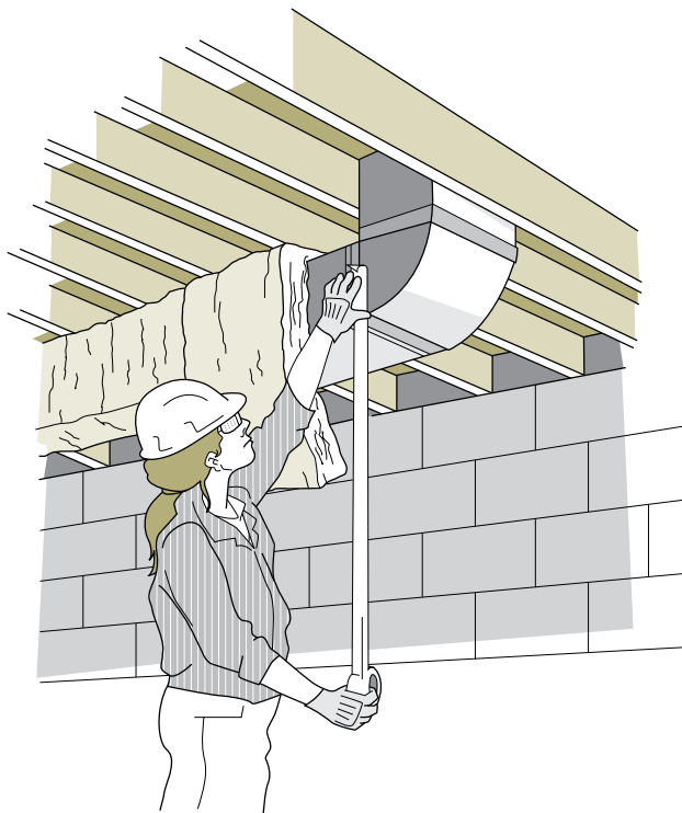
Figure 9-1 Taping an air duct
