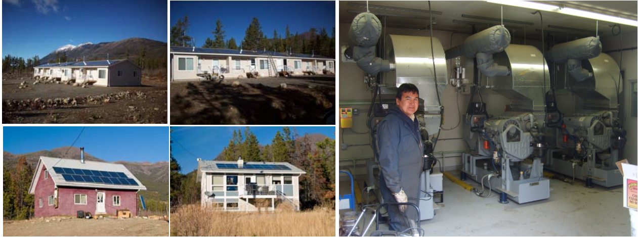
Figure 4: Residential PV systems and diesel gensets supplying the Nemiah Valley mini-grid (Credit: Dave Turcotte and Andrew Swingler).
