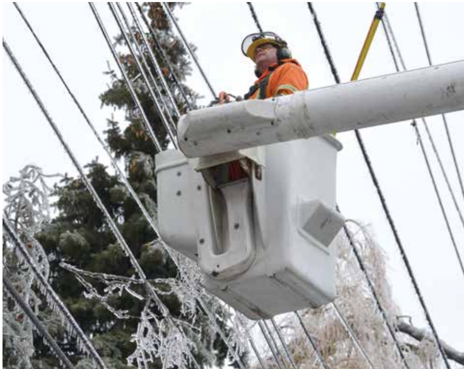
Toronto Hydro Corporation's linesman in a bucket truck during the 2013 ice storm. The storm ravaged the City of Toronto over the winter holiday season. Photo courtesy of Toronto Hydro Corporation.
