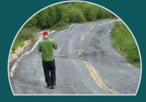
The frozen ground, called permafrost, in Canada's north is warming, which can cause the land to sink, damaging buildings, roads and other infrastructure.
