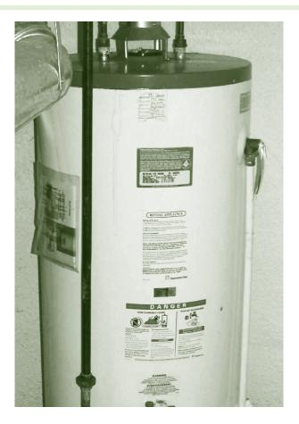
The standard gas-fired water heater is called a conventional or naturally aspirating water heater. Its tank is
