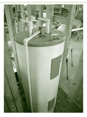
The tank of an electric storage tank water heater is
