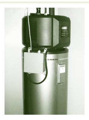
**Heat pump water heaters** (HPWHs) use electricity to transfer heat from the air instead of converting electricity directly to heat. Heat is taken from the air in the basement or utility room (or sometimes from outside) and transferred to a tank of water. HPWHs remove heat and humidity from the air. As heat is removed from inside the home in summer, you will need less air conditioning. HPWHs are less advantageous in the winter when space heating is required.
