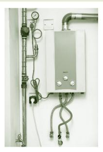
This type of water heater consists of either an electric element or a gas burner that heats flowing water and does not have a storage tank. It is also called on-demand, point-of-use, instantaneous or tankless water heater because it heats water only when it is needed, thereby eliminating continuous standby losses. A tankless water heater is usually more energy-efficient than a storage tank water heater.
