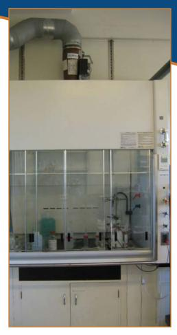
New high efficiency/low airflow fume hood
