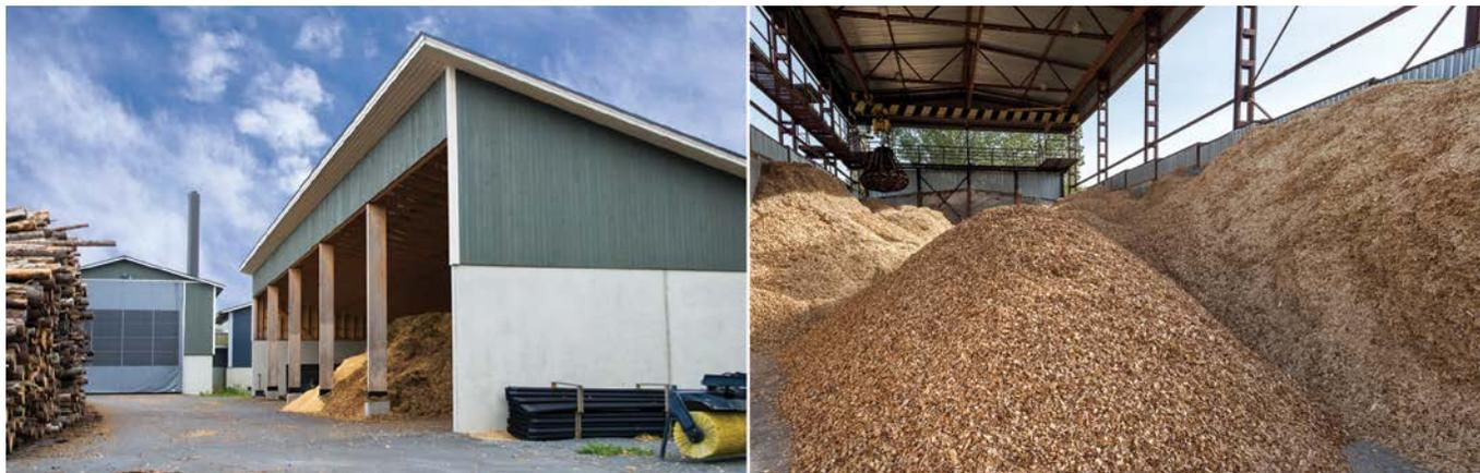
**Figure 2.** Covered storage for wood chip piles
