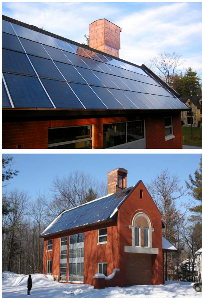
Figure 2: The Alstonvale Net Zero Energy House, Hudson, Quebec, Canada. (Photos credits: Sevag Pogharian)
