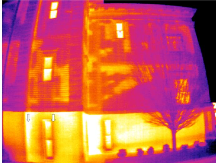
Figure 4: Thermal image of front building envelope, showing missing insulation (Sagewell)<sup>53</sup>
