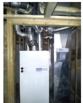
Zoned air handler installation
