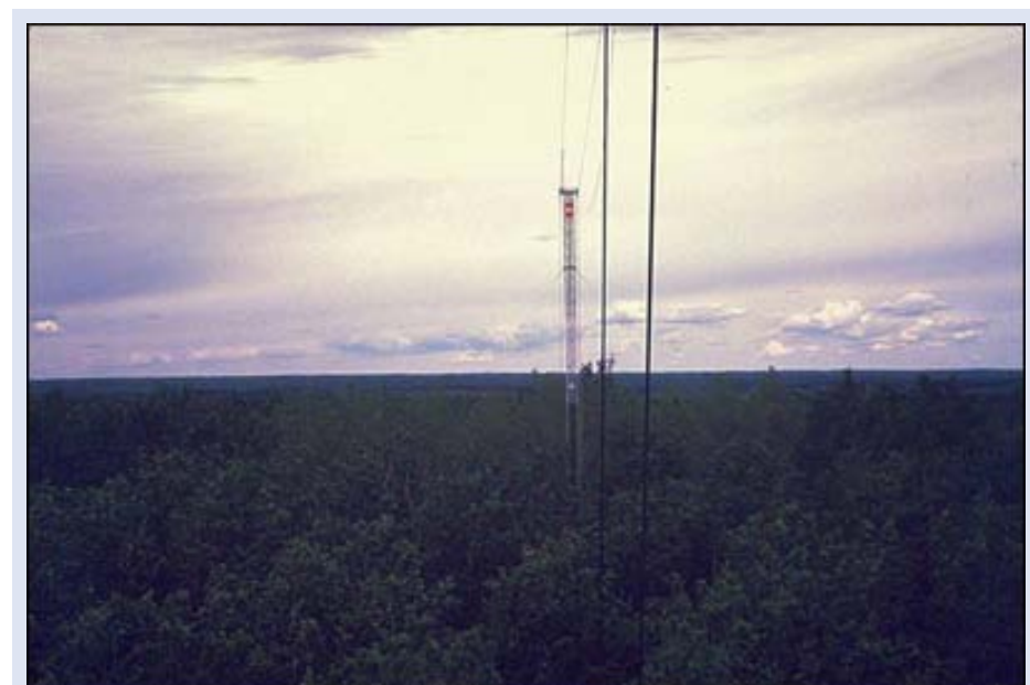
Figure 2. Flat tower in Prince Albert National Park
